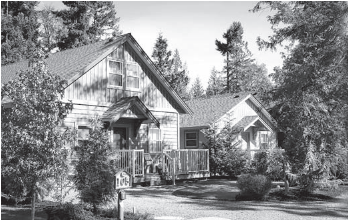
Plans for phase two of the Oceanside Village Resort on Vancouver Island include vaulted ceilings. SHOREWATER ESTATES LTD.
